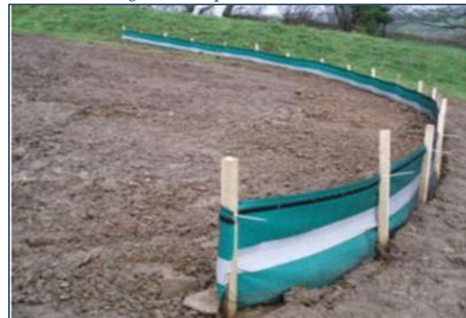
Plate 3-4. Embedded Silt Fence
